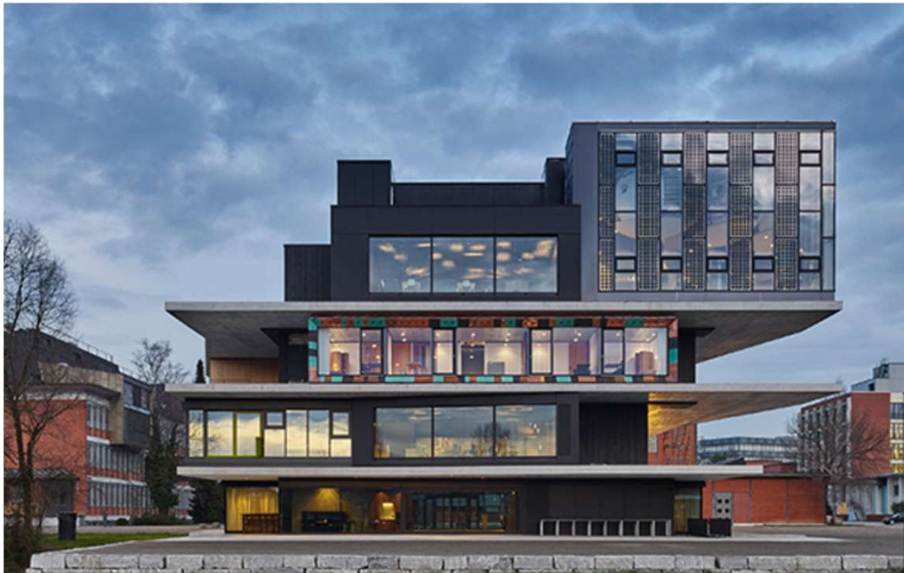
Example of the NEST infrastructure in Switzerland
